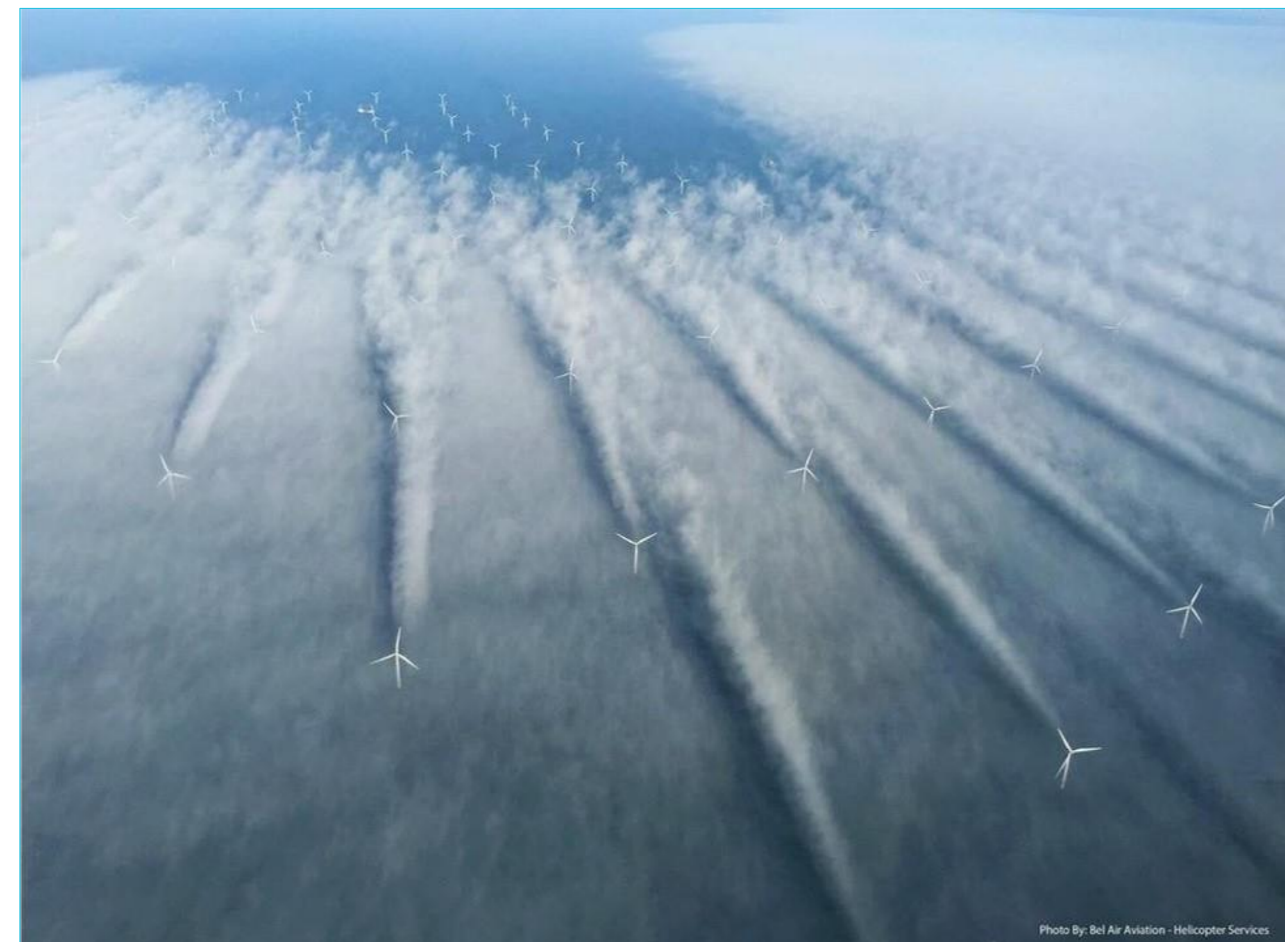
↑ Horns Rev 2 offshore wind farm in fog showing wake effects. Photo 3 particularly highlights the increased turbulence caused by upwind turbines. These turbines are 2.3MW.
