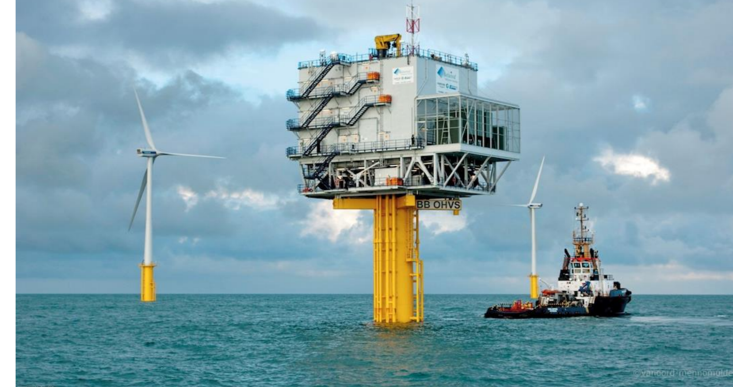
Mainstream’s NEART NA GAOITH SUBSTATION:
