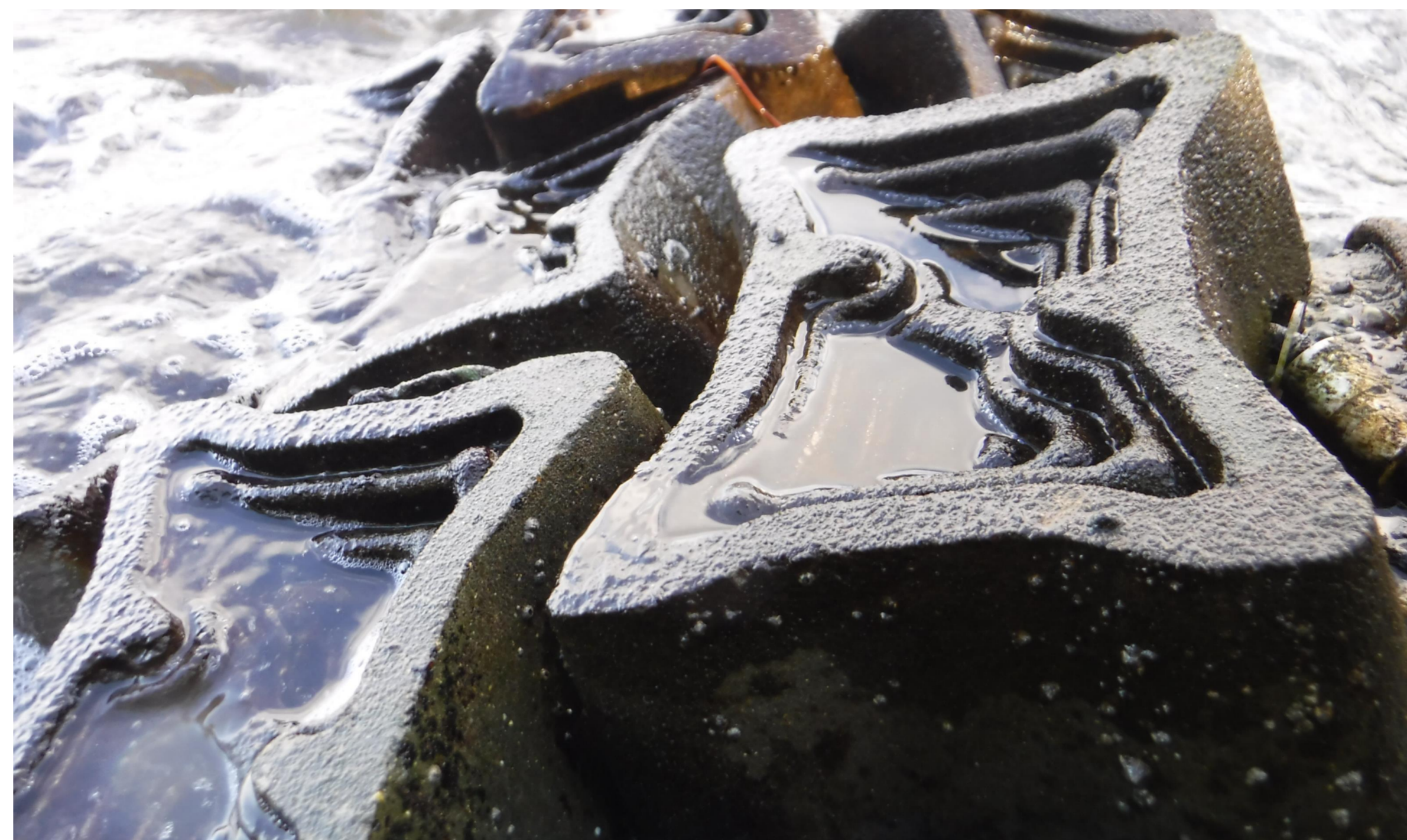
ECO ACBM retaining water as the water level recedes, providing tide pool habitat
