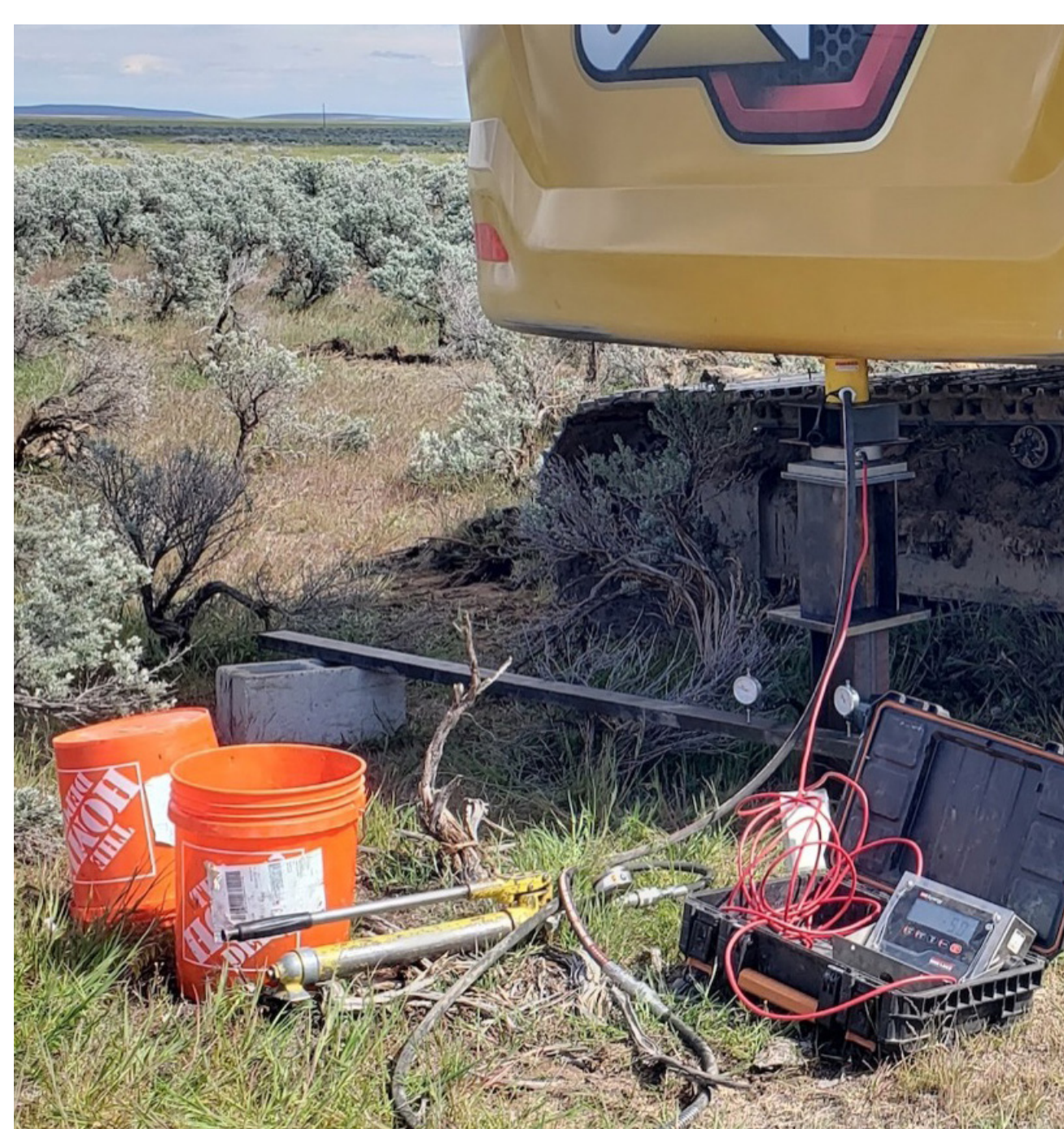
Compression pile load testing using excavator.
