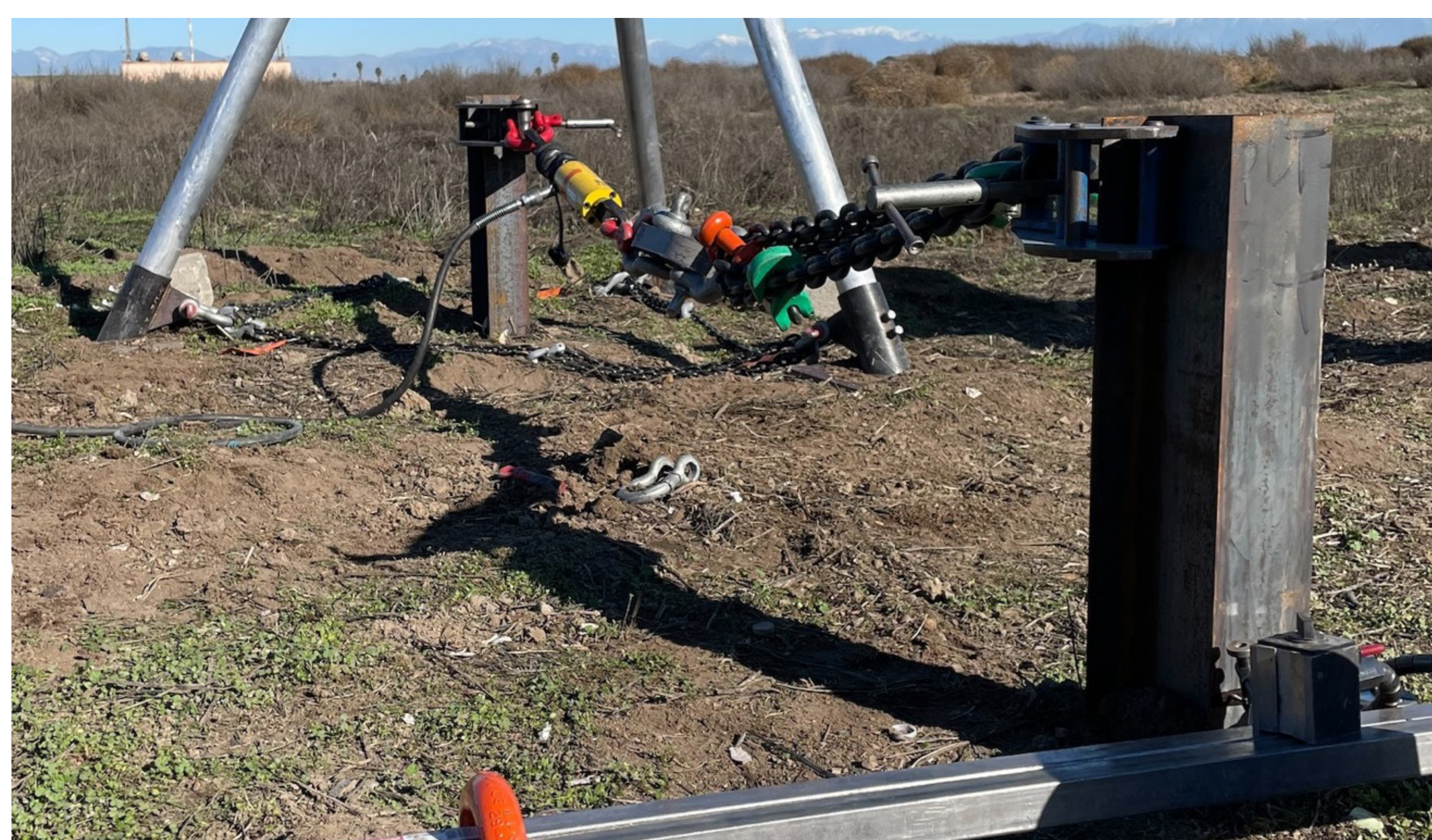
Lateral pile load testing with the hydraulic jack.
