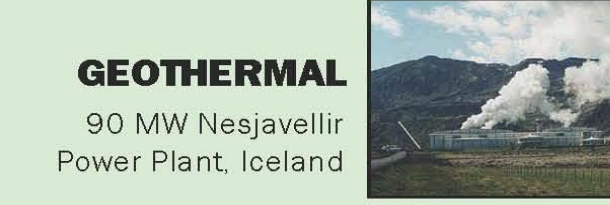
GEOTHERMAL 90 MW Nesjavellir Power Plant, Iceland
